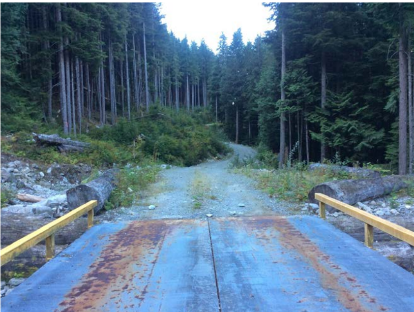
Left approach viewed from bridge
