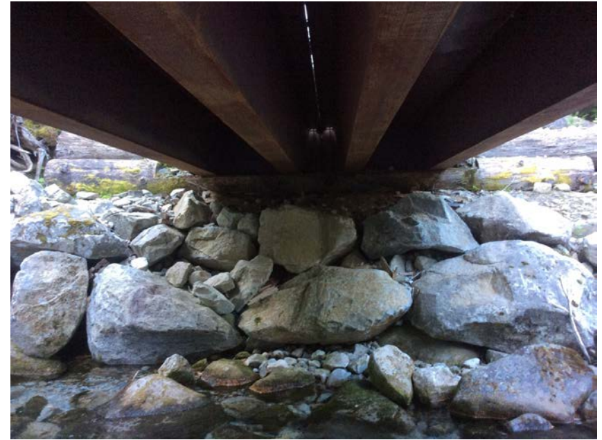
Left Bank Abutment when facing downstream
