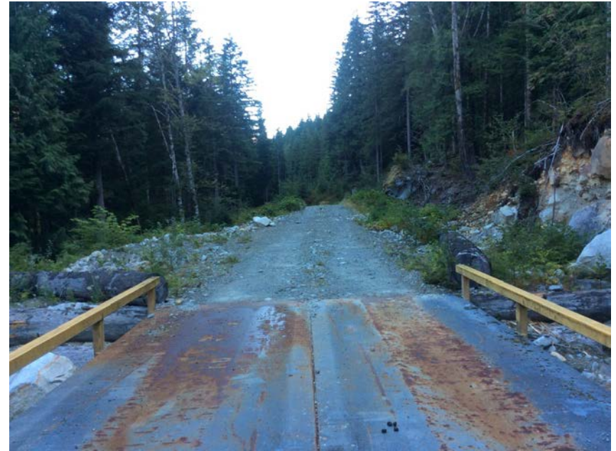
Right approach viewed from bridge
