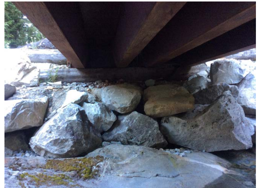
Right Bank Abutment when facing downstream
